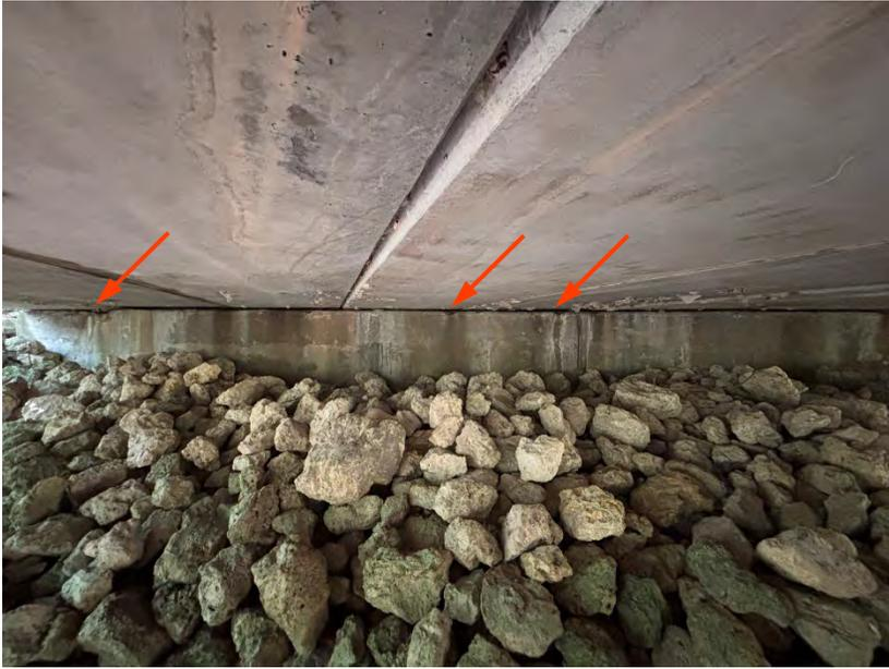
PHOTO 11 – ABUTMENT 1, EDGE SPALLS, CRACKS
