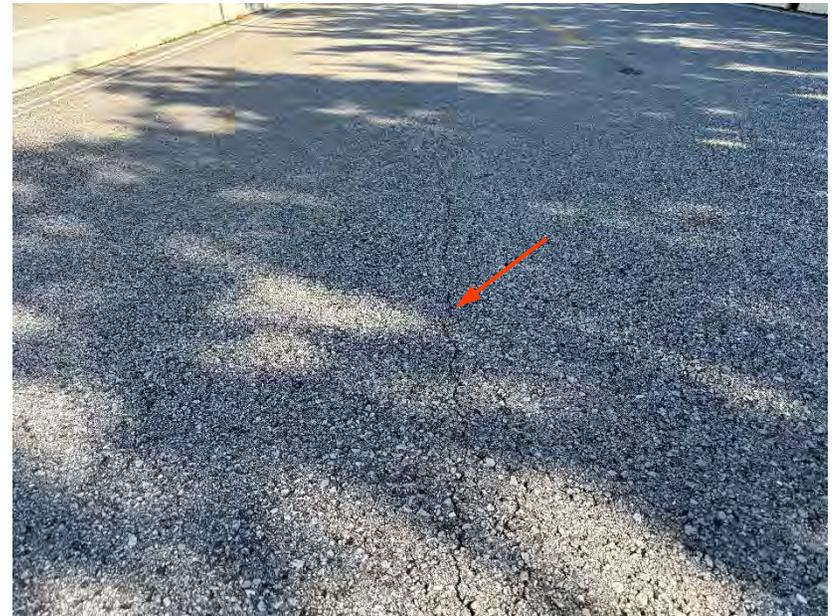
PHOTO 4 – TYPICAL ASPHALT CRACKING
