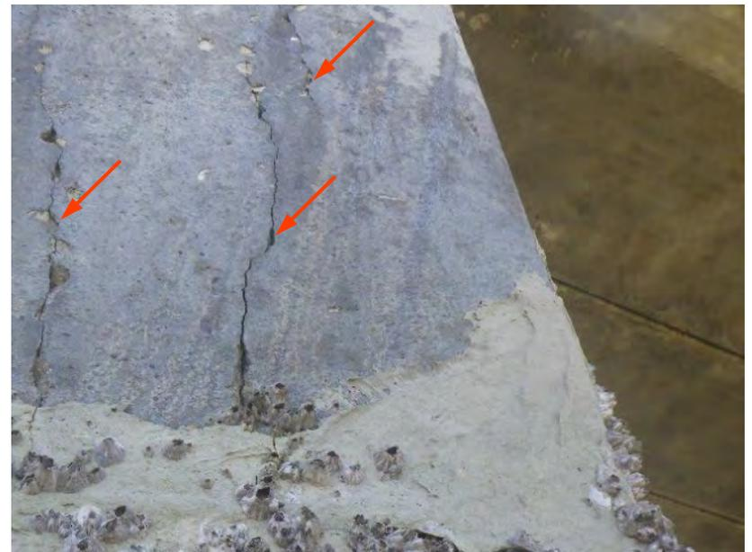
PHOTO 14 – PILE 9-6, VERTICAL CRACKS
