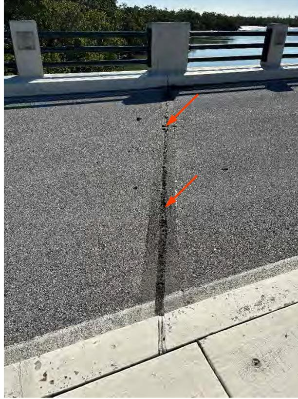
PHOTO 9 – EXP. JT. 11, ADHESION FAILURE, RUTTING
