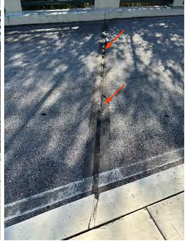
PHOTO 10 – EXP. JT. 14, ADHESION FAILURE, RUTTING
