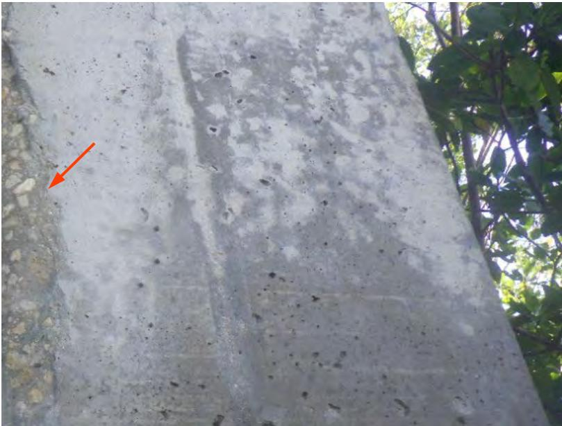
PHOTO 13 – PILE 7-1, EDGE SPALL
