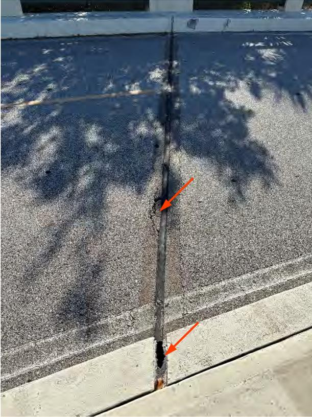
PHOTO 5 – EXP. JT. 1, ADHESION FAILURE, RUTTING
