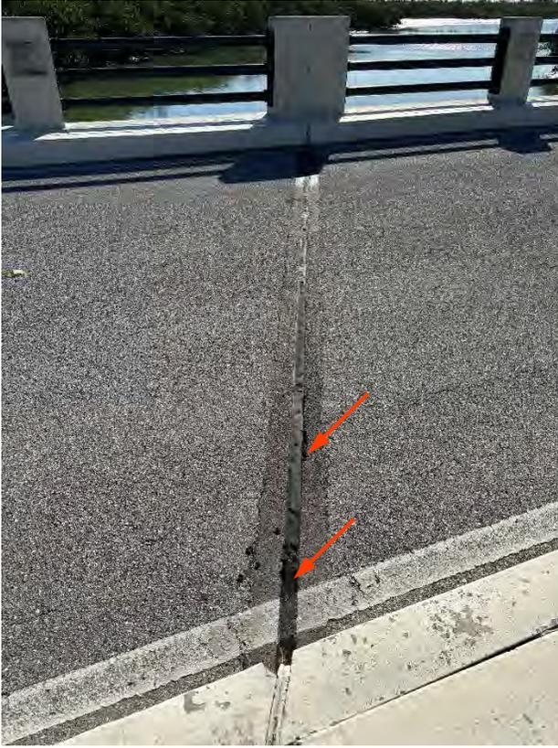
PHOTO 8 – EXP. JT. 9, ADHESION FAILURE, RUTTING
