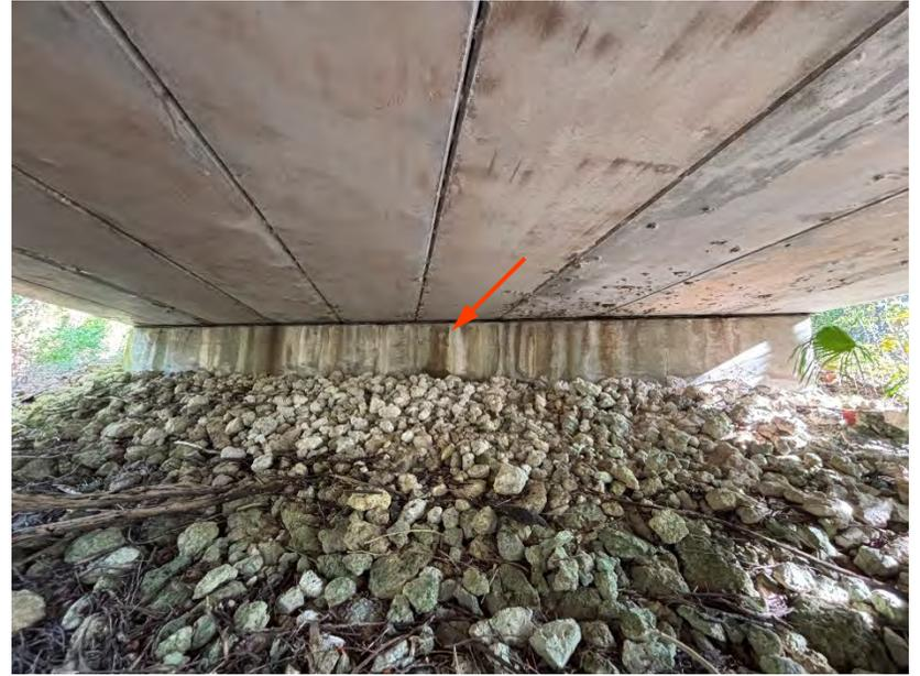
PHOTO 12 – ABUTMENT 14, JOINT LEAK STAINS
